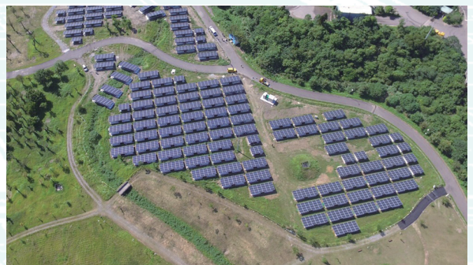
Solar PV system at Shanshailu Eco Park in Nangang
