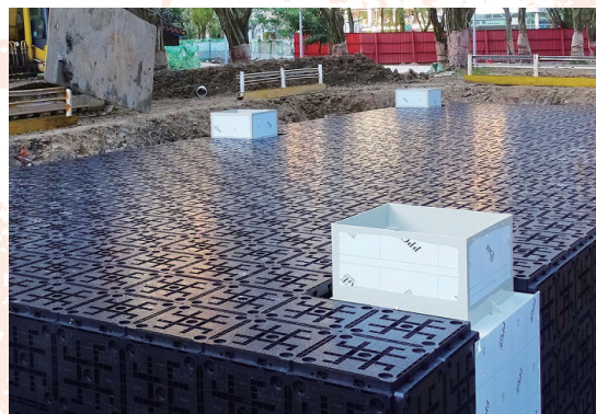
A brick-type rainwater harvesting facility in Xiangshan Park
