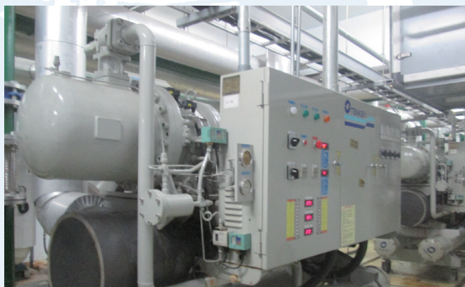
Neihu Precinct, Taipei City Police Department: Inspection of central air-conditioning unit
