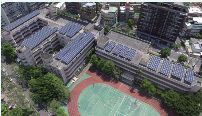
Solar PV system at Lanya Elementary School
