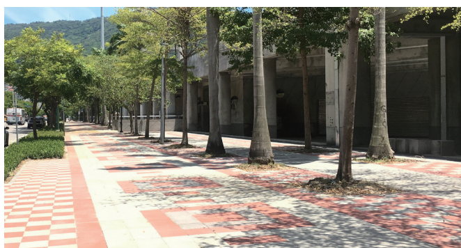
Permeable pavements on the sidewalks around Tianmu Baseball Stadium
