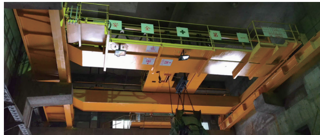
Refurbishment of ash-handling crane with a new operation room
